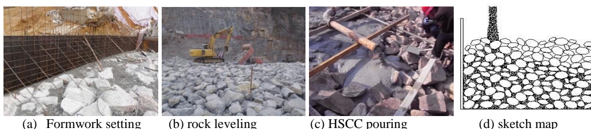
Figure 1: construction process and sketch map of Rock-Filled Concrete
