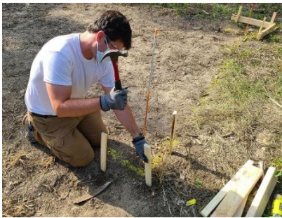
Figure 6. Installing Batter Boards
