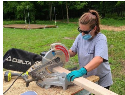
Figure 7. Cutting for Batter Boards
